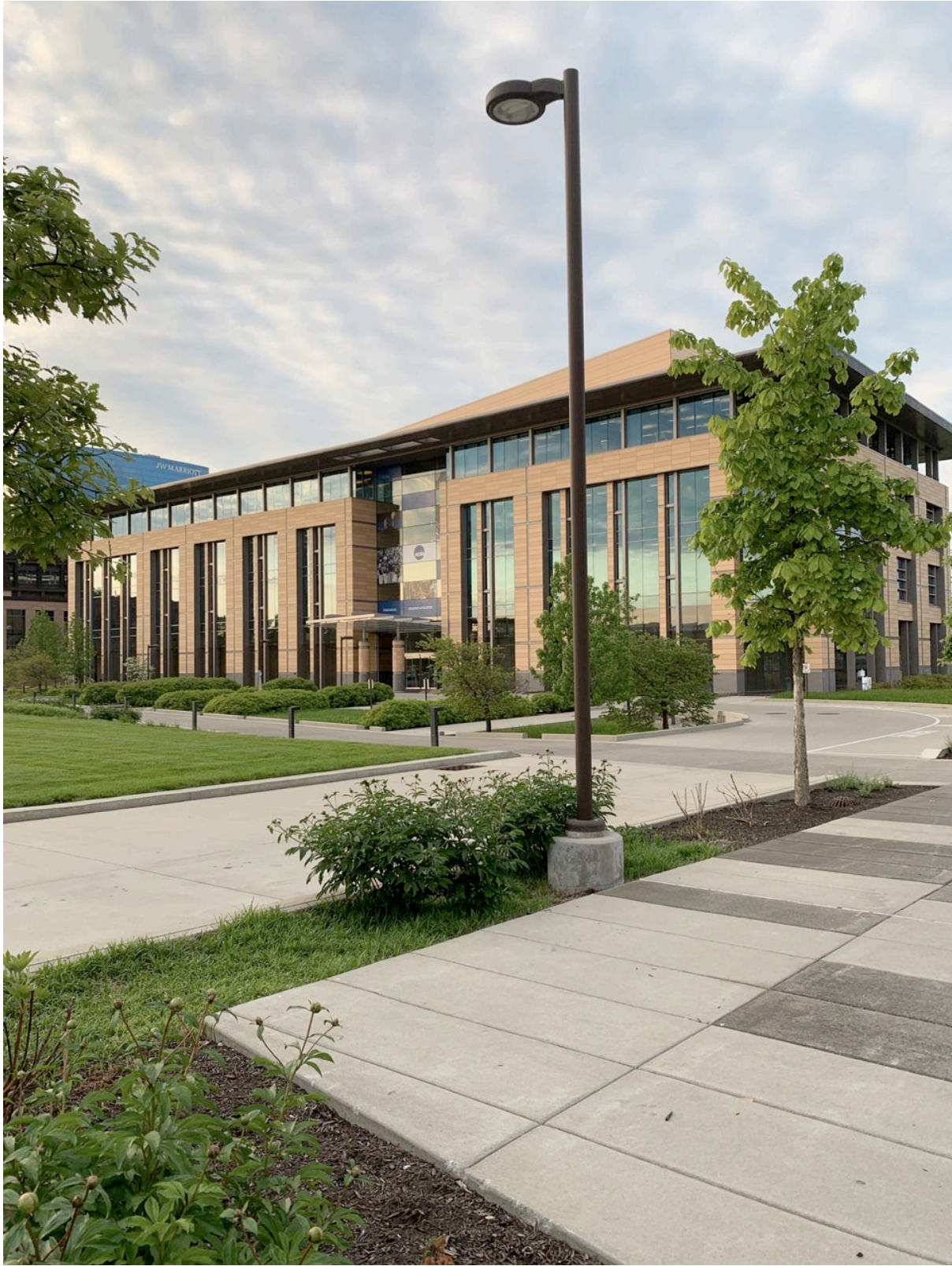
Myles Brand Headquarters Building, NCAA, Indianapolis, IN
